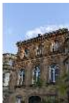
BayFa.I, Nordfassade (Detail), DI017167, BSV-
