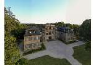
BayFa.I, Nordfassade, DI017100, BSV-
