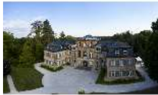
BayFa.I, Nordfassade, DI017107, BSV-
