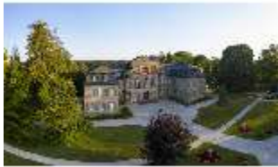
BayFa.I, Nordfassade, DI017106, BSV-
