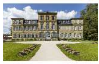
BayFa.I, Südfassade, DI002641, BSV
