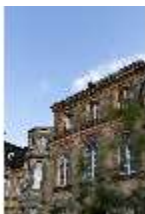
BayFa.I, Nordfassade (Detail), DI017166, BSV-
