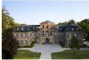
BayFa.I, Nordfassade, DI017098, BSV-
