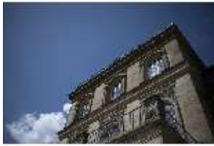
BayFa.I, Fassade (Detail), DI017158, BSV-
